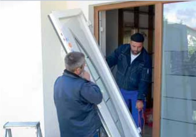
Step 2: The new Hörmann entrance door is fitted by the authorised Hörmann partner according to the measurements. The special entrance door threshold neatly covers up the transition from the interior to the exterior. The doors are fixed to the ground by concealed screws.
