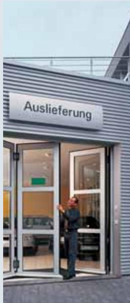
**3** Folding doors made of steel and aluminium
